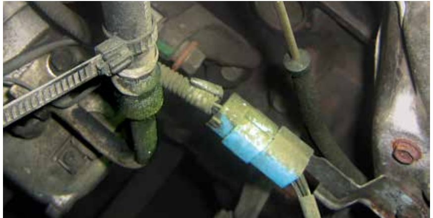
This 2004 Frontier lost its refrigerant recharge over the course of a week. Thankfully, this leaking high pressure hose was easy to identify.
